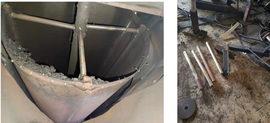
Figure 3. 2 The condition after the replacement of the shaft support component.
