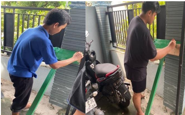
Gambar 1. Pengecatan rambu himbauan peringatan
