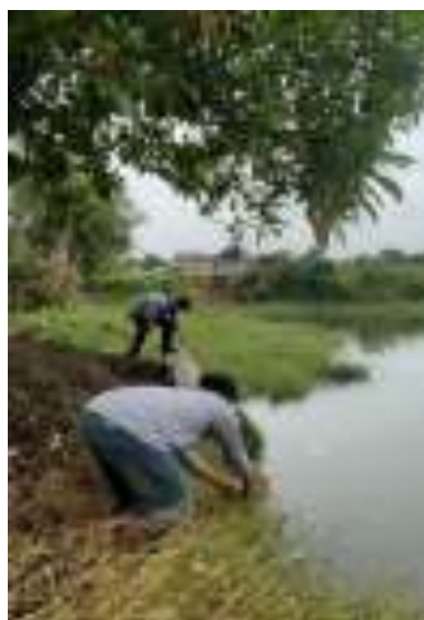
Gambar 4. Survei Lokasi Dinding Penahan Tanah
