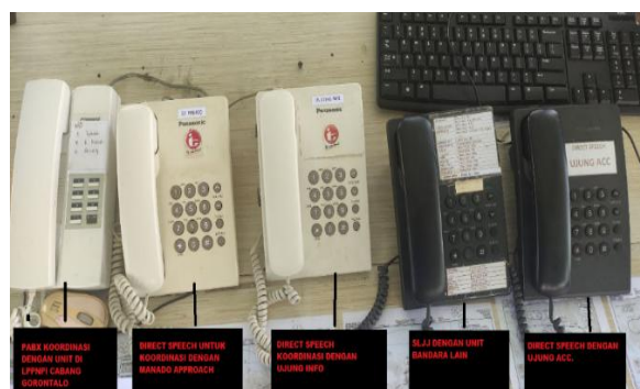
Figure 2. Coordination Unit Djalaluddin Tower
