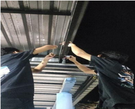
Figure 1. Team KKN do installation photocell
