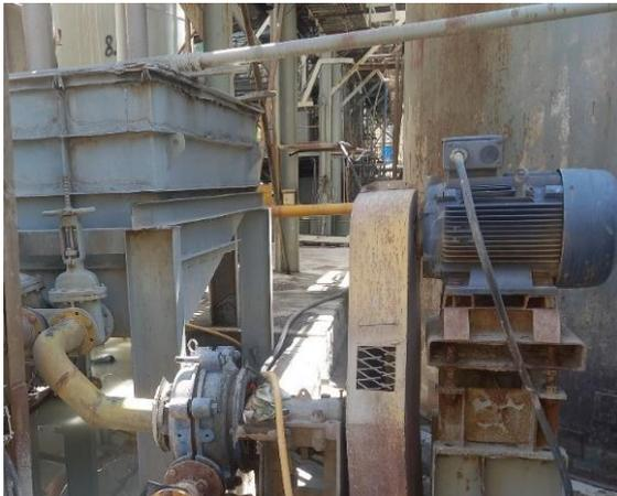
Gambar 2. Pompa sentrifugal tipe 6/4 D-AH
