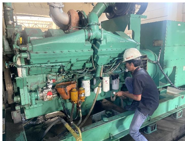
Gambar 5. Maintenance sistem pendingin mesin diesel Cummins KTA 38 G5
