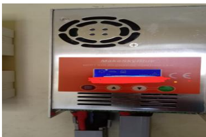
Gambar 2. BCR (Battery Control Regulator)
